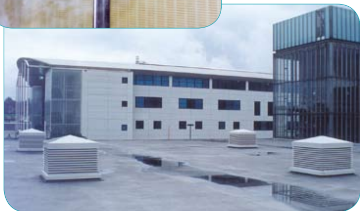
Below: Windcatcher units installed on flat roof of old central mainframe computer building
